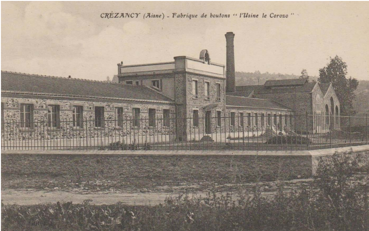
Figure 3. Corozo factory in Crézancy
